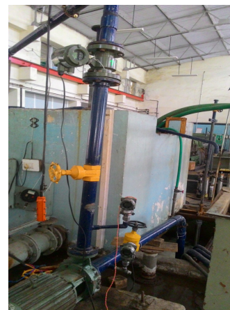
Fig. 5. Centrifugal pump performance test setup as per ISO 9906.
