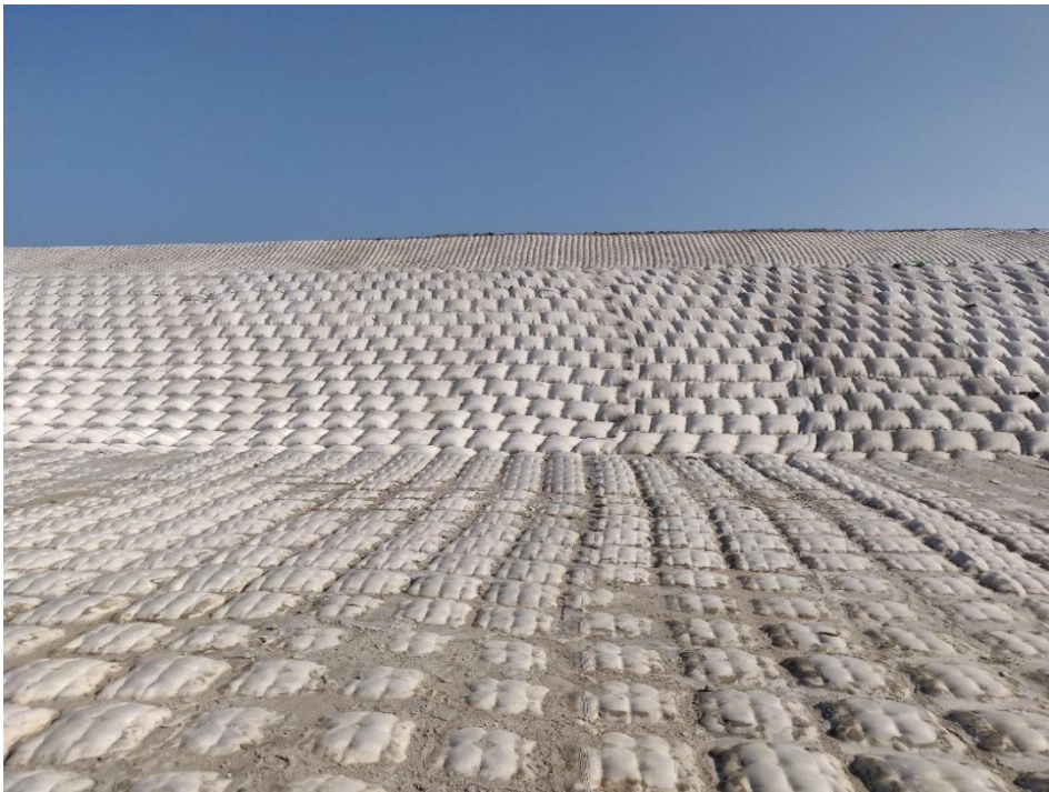
Figure 4. Articulating Block Concrete Mattress after installation at site
