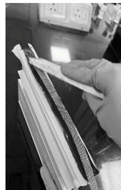
d) WIRE MESS SCREEN BEING IMBEDDED IN WET SEALANT BEAD
