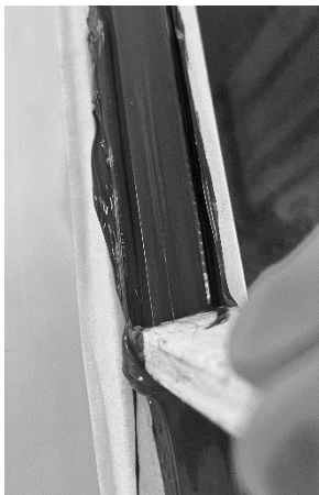
g) TOOLING SECOND BEAD OF SEALANT WITH SPECIAL TOOLING DEVICE — SIDE B
