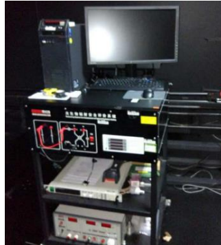
Fig 23 Power Supply Unit
