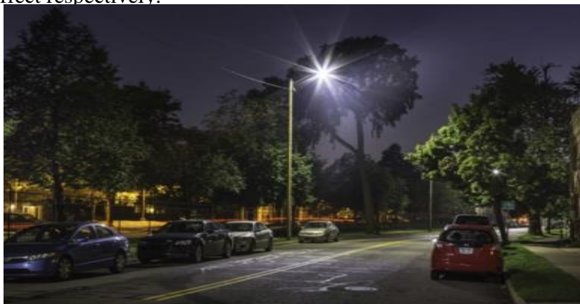
Fig. 6 Street Lighting Glare
