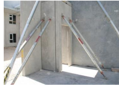
FIG. 9 PROP FOR PRECAST STRUCTURE
