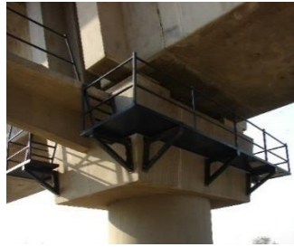
FIG. 8 FIXING OF WALKWAY
