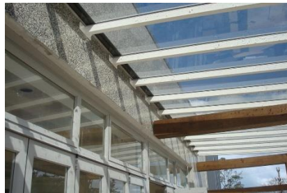
FIG. 3 FIXING OF BRACKET FOR CANOPY AND SKYLIGHT
