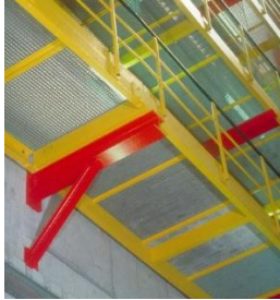
FIG. 8 FIXING OF WALKWAY
