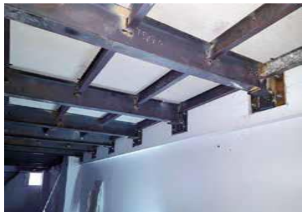
FIG. 5 FIXING OF BRACKET FOR MEZZANINE FLOOR
