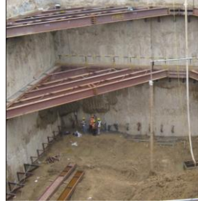
FIG. 7 FIXING OF STRUT WALER
