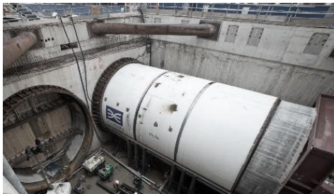
FIG 11. FIXING OF KICKER-RING DURING TBM LAUNCH
