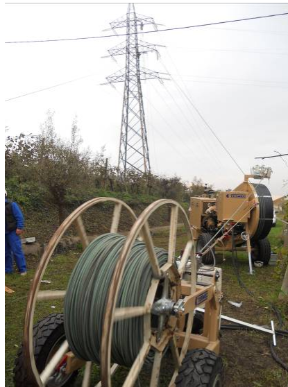
a) Drum puller, two single drums (IEC 60743)
