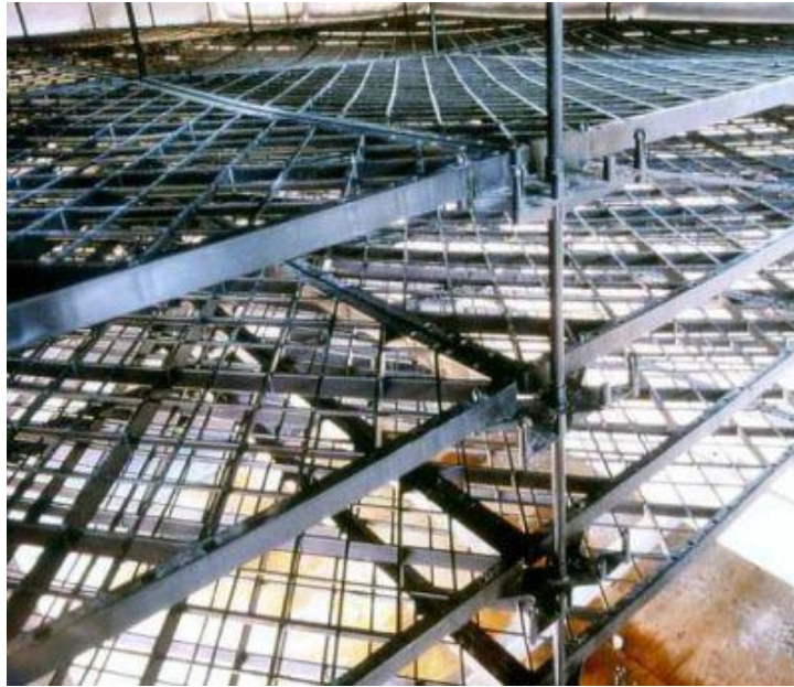
FIG. 5A PP SPLASH GRID
