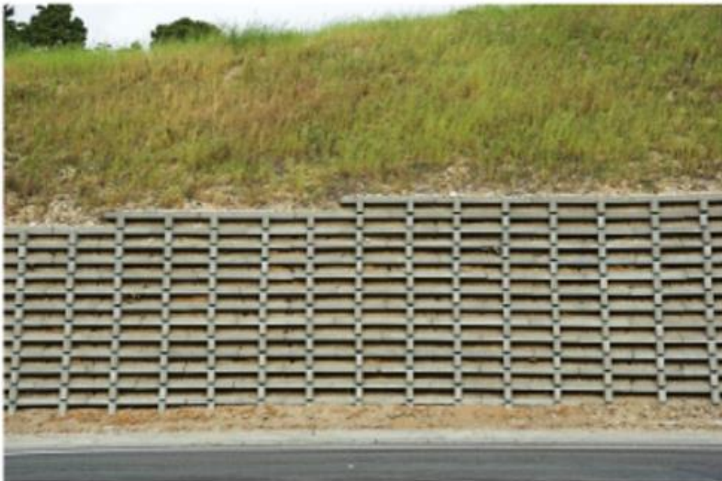
FIG. 8 CONCRETE CRIB WALL
