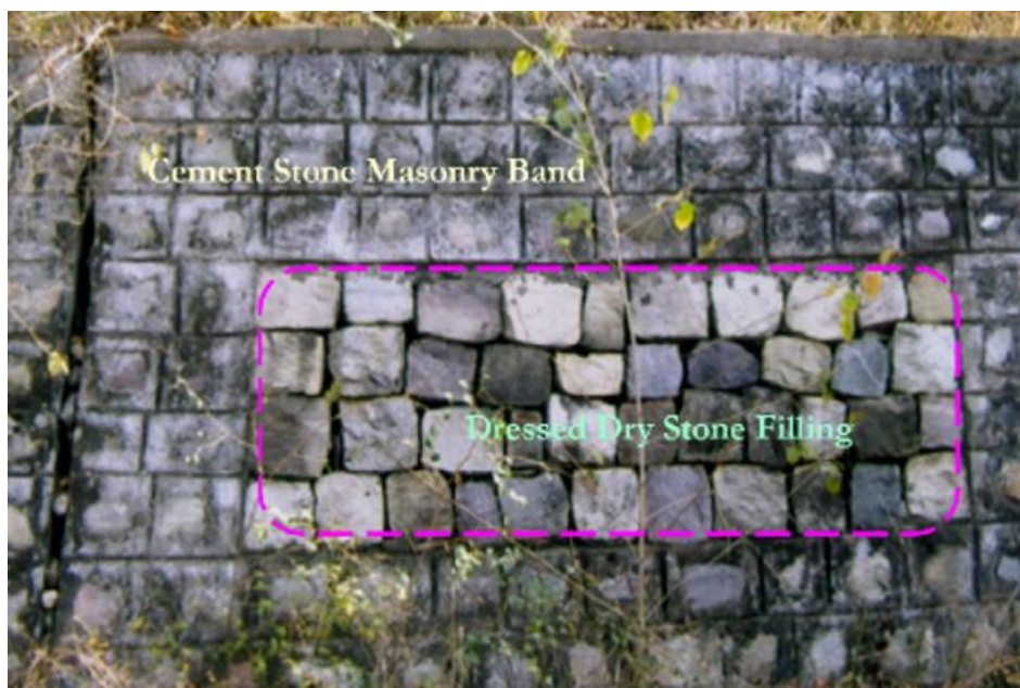
FIG. 11 BANDED STONE MASONRY WALL
