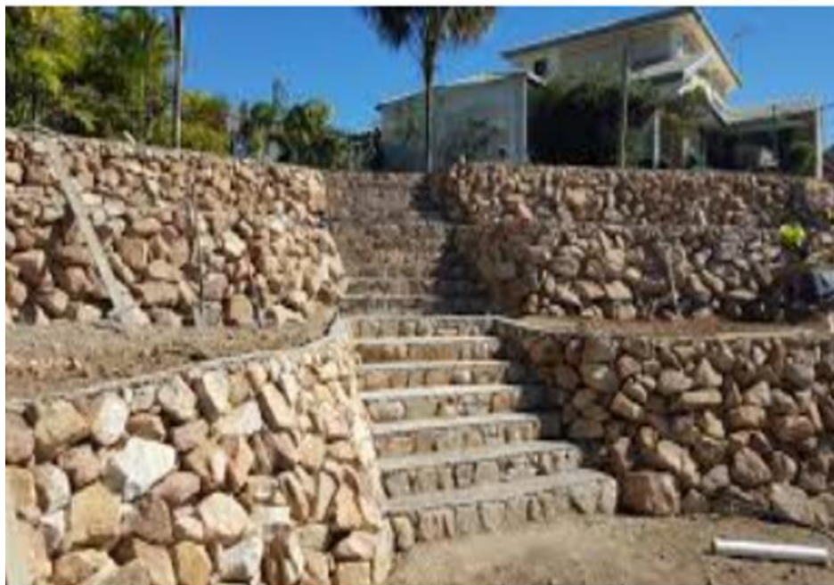
FIG. 10 DRY STONE RETAINING WALL
