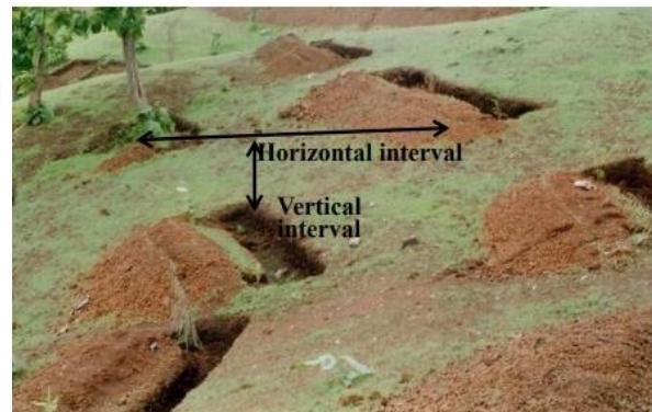
FIG. 14 SCHEMATIC AND PICTURE OF A STAGGERED CONTOUR TRENCH
