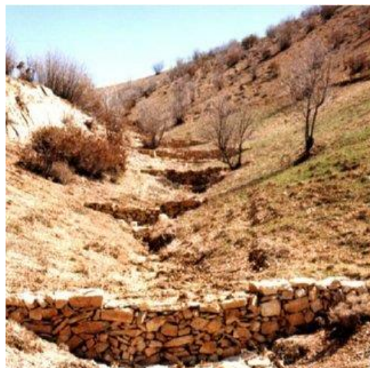
FIG. 12 SCHEMATIC AND PICTURE OF A LOOSE STONE CHECK DAM
