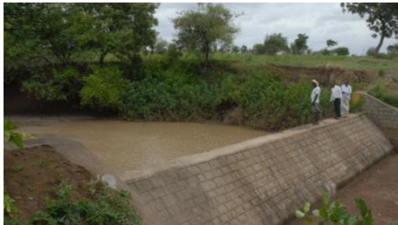
FIG. 10 PHOTOGRAPHIC VIEW OF A TYPICAL CHECK DAM
