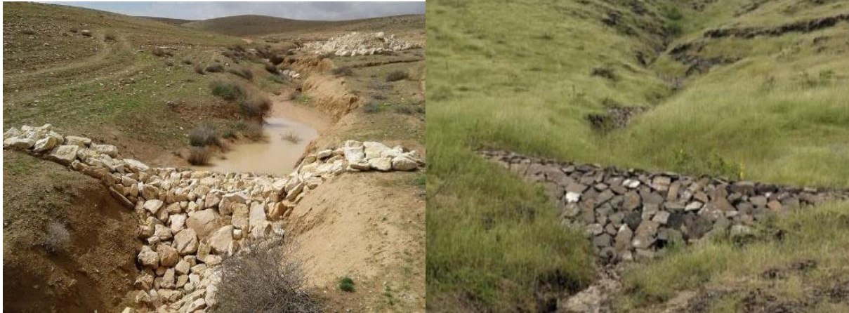
FIG. 16 PHOTOGRAPHIC VIEW OF TYPICAL GULLY PLUGS
