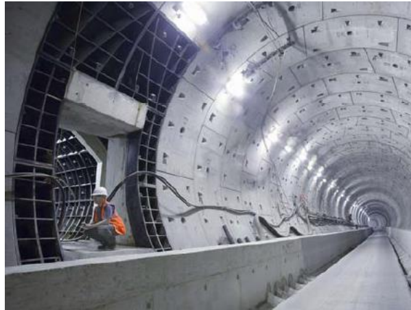
FIG. 11 PREFABRICATED STEEL SEGMENTS
