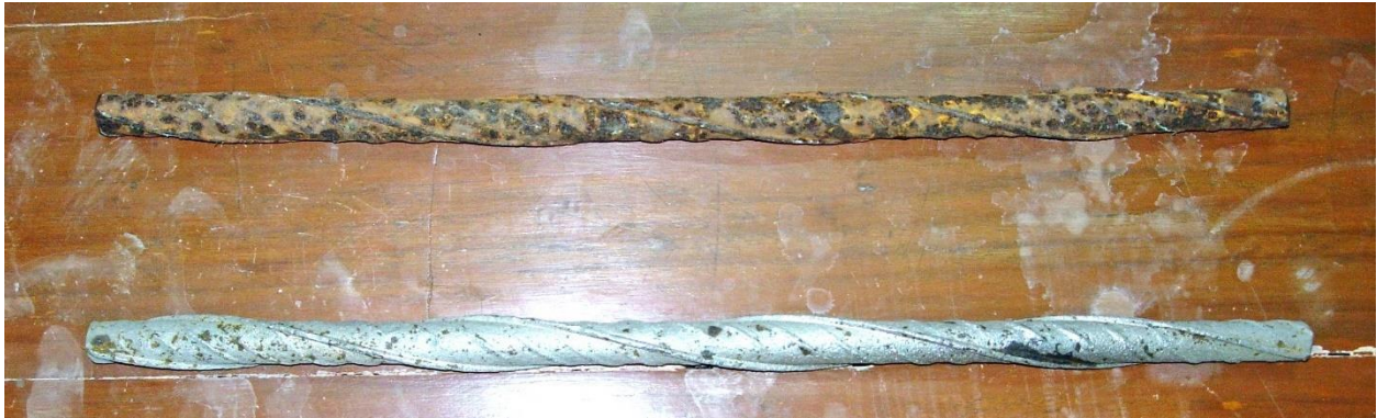
Figure 19 Corroded steel rebar cleaned to determine the cumulative corrosion rate
