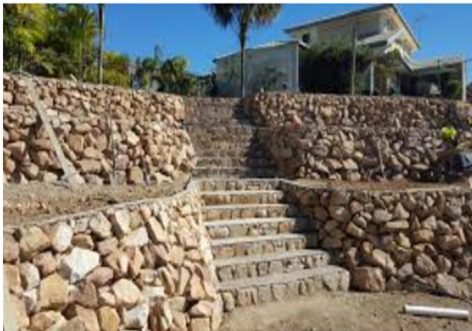
FIG. 10 DRY STONE RETAINING WALL
