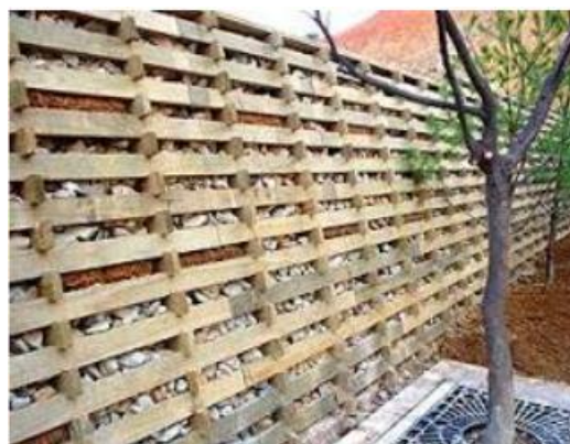
FIG. 14 A TIMBER CRIB RETAINING WALL
