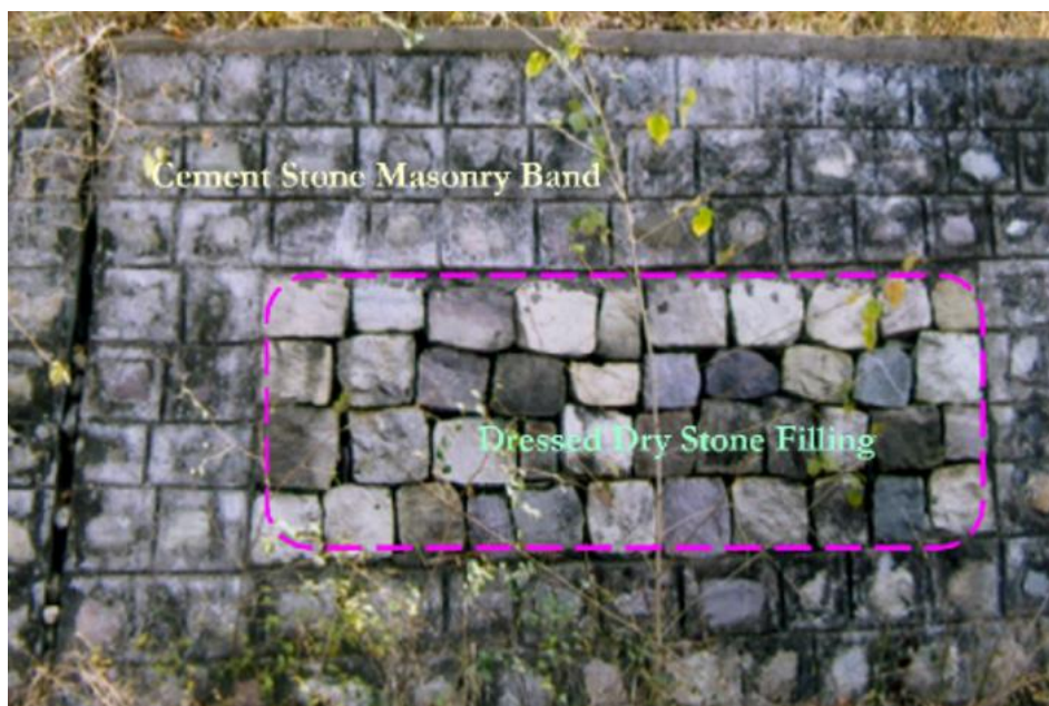
FIG. 11 BANDED STONE MASONRY WALL
