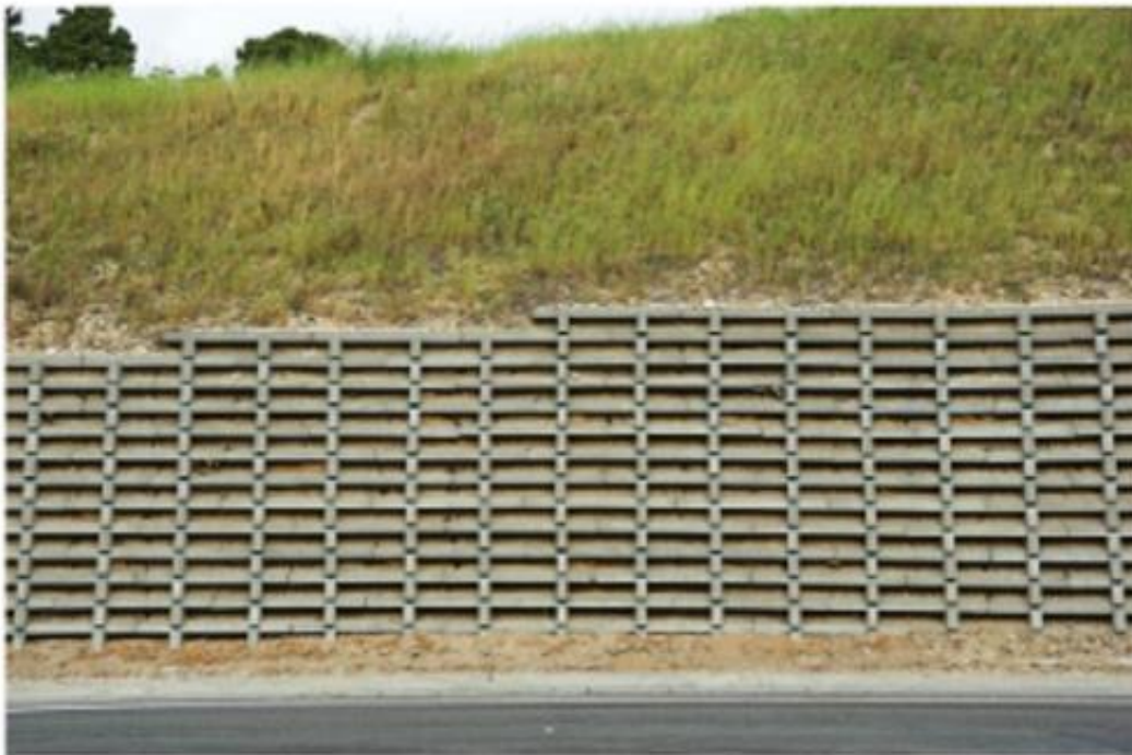
FIG. 8 CONCRETE CRIB WALL
