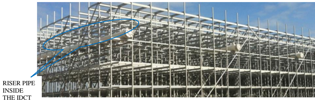
FIG. 9 INDICATIVE IDCT CROSS-SECTION (FRP TOWER)
