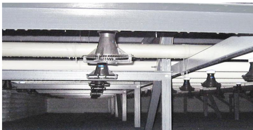
FIG. 10 INDICATIVE DISTRIBUTION PIPES PLACED ABOVE BEAMS
