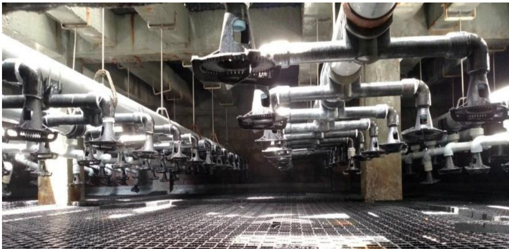
FIG. 11 INDICATIVE DISTRIBUTION PIPES FIXED BELOW RCC BEAMS
