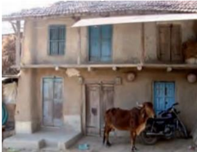
FIG. 1 COB WALL HOUSE IN PANDAD VILLAGE, ANAND, GUJRAT
