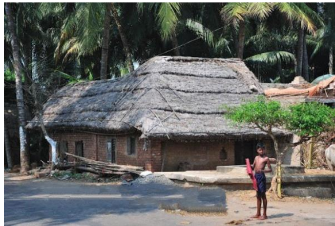
FIG. 13 BRICK MASONRY WALLS WITH HIPPED THATCHED ROOF
