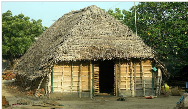
FIG. 20 WOOD AND BAMBOO WALL WITH THATCHED ROOF
