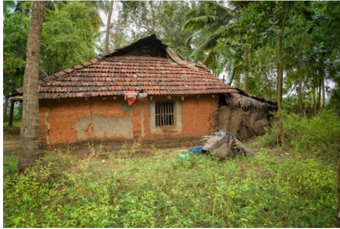
FIG. 10 MUD WALLS WITH TILED ROOF
