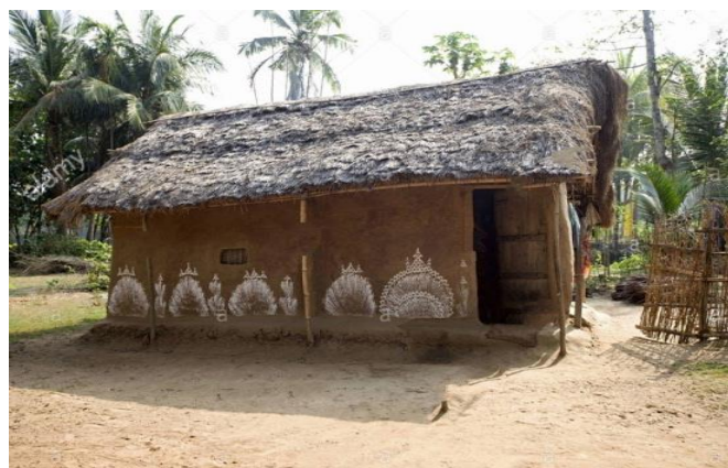
FIG. 9 MUD WALL AND THATCHED ROOF HOUSE, PURI, ODISHA
