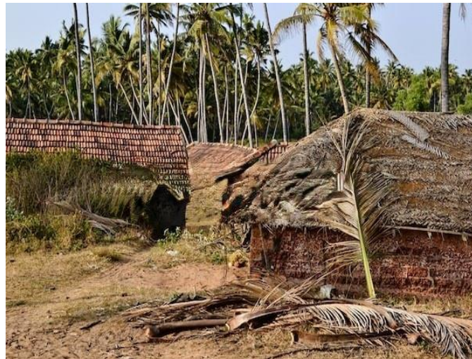
FIG. 19 THATCHED AND TILED ROOF WITH STONE MASONRY WALLS
