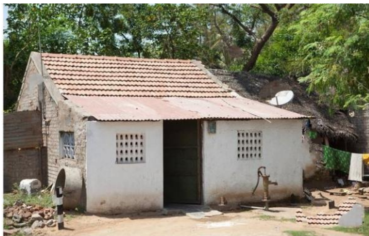
FIG. 14 BRICK MASONRY WALLS WITH TILED AND CGI SHEET ROOF
