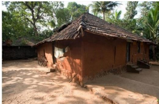
FIG. 8 MUD WALLS WITH TILED ROOF RATNAGIRI, MAHARASHTRA
