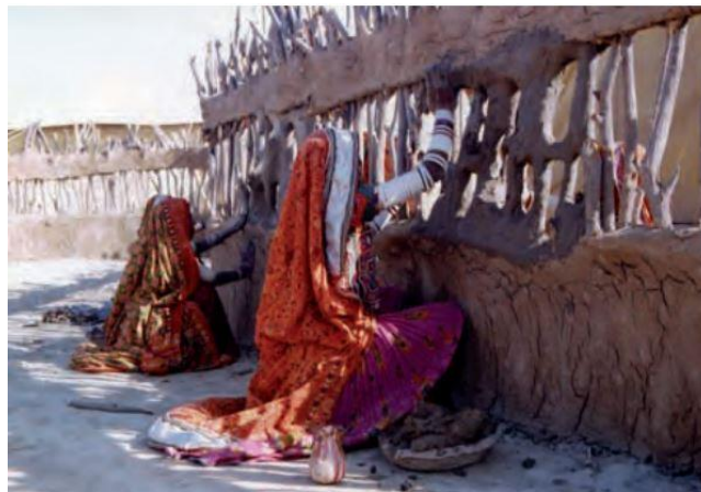
FIG. 6 DAUB IS APPLIED FIRMLY OVER THE LATTICE BY WOMEN
