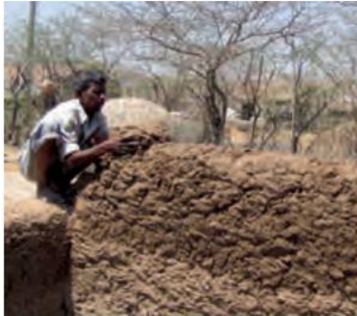
FIG. 2 COB WALL CONSTRUCTION
