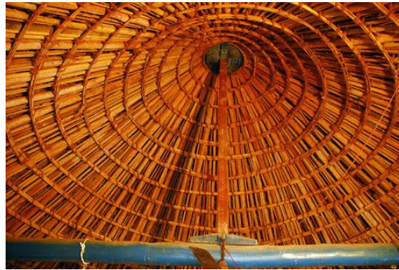
FIG. 22 BHUNGA HUT AND THEIR CONICAL ROOF INSIDE VIEW
