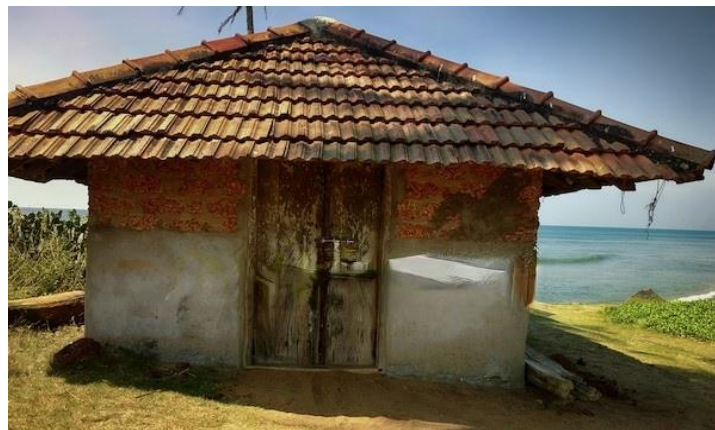
FIG. 17 LATERITE STONE MASONRY WALL WITH TILED ROOF
