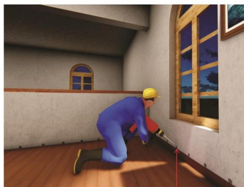
Drilling at 300mm distance above skirting
