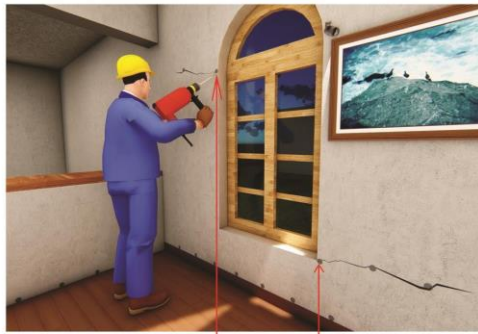
Drilling holes at voids and cracks
