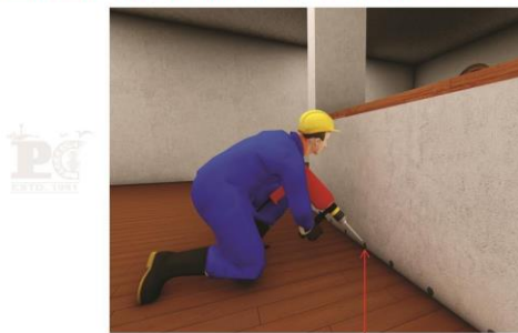
Drilling at 300mm distance for junction of wall and floor (without skirting)
