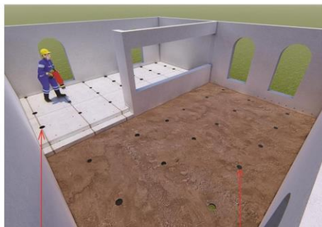
Drilling holes for existing flooring
